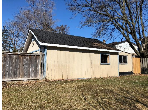
Image 15: View northwest towards garage
