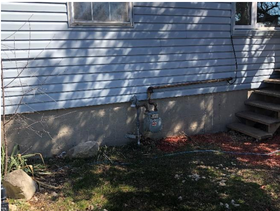
Image 11: View towards the foundation on south side elevation
