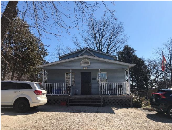
Image 3: View southeast at front elevation
