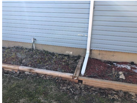
Image 8: View at foundation join on north side elevation
