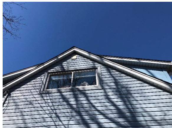
Image 6: View at second storey window and roofline of rear elevation
