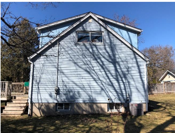
Image 5: View west toward rear elevation
