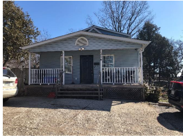
Image 4: View east at front elevation
