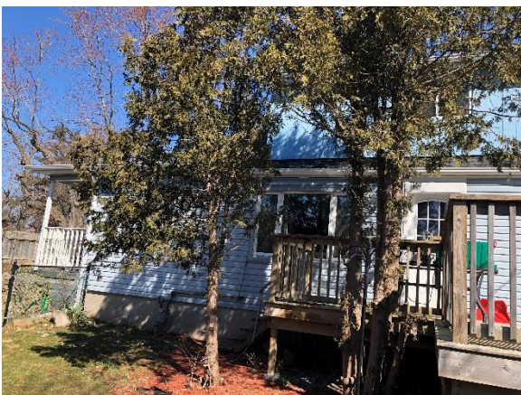
Image 13: View of door on south elevation and wooden deck
