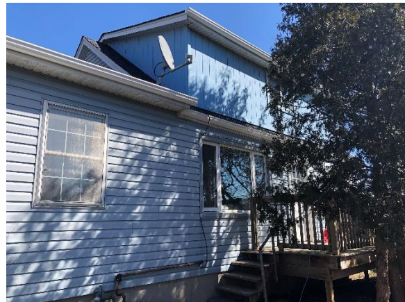
Image 12: Looking northeast at south side elevation
