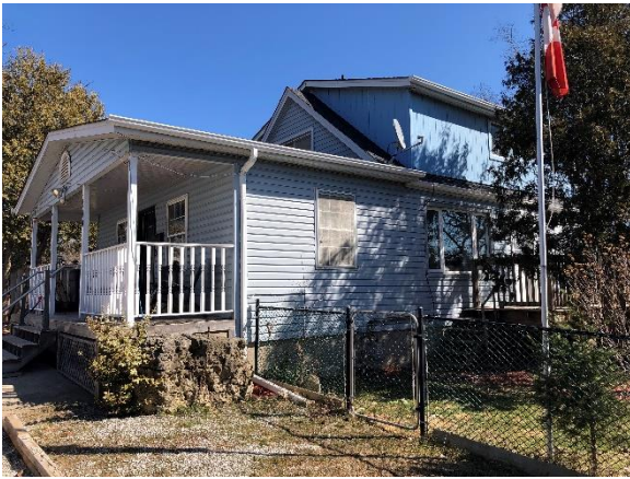
Image 9: View northeast toward south side elevation
