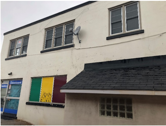
Image 15: View northwest of south elevation.
