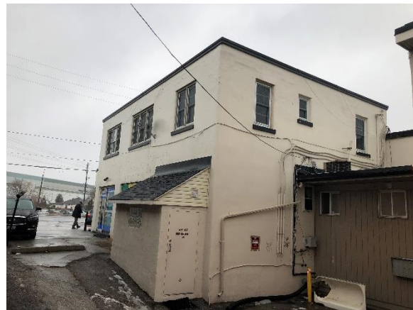
Image 14: View northwest of south and east elevation.
