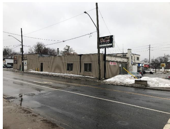
Image 12: View southeast of north elevation.
