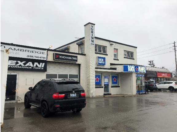
Image 7: View east of stucco garage attached to two-storey structure.
