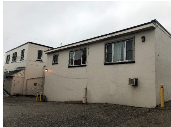
Image 16: View northwest of south elevation.
