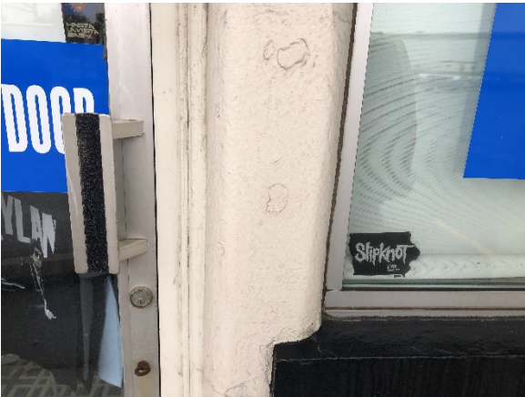
Image 6: View of curved stucco on the window and door openings.
