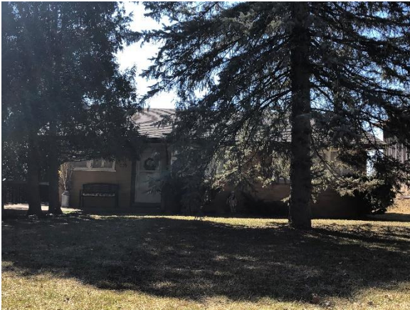
Image 7: View of front elevation, note recessed entrance
