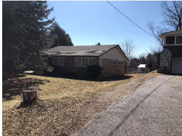
Image 8: View of west side of front elevation
