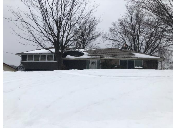
Image 4: View of front (north) elevation
