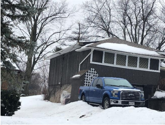
Image 5: View of the east side elevation
