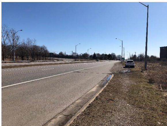
Image 11: View looking generally southeast of the subject structure
