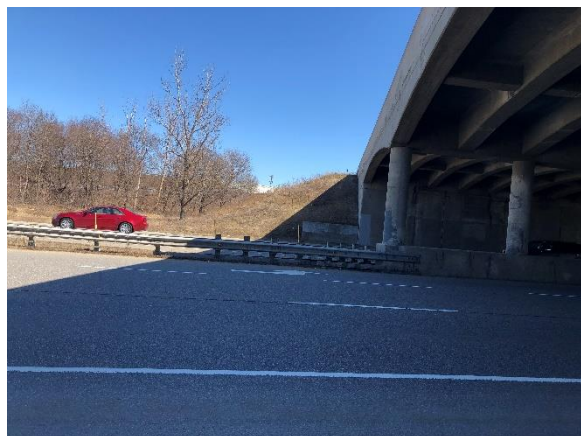
Image 8: View east along the north elevation of the structure
