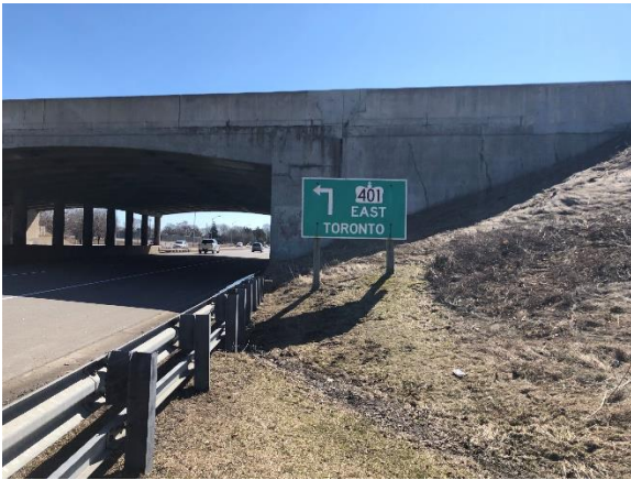
Image 3: View south of the northwest abutment
