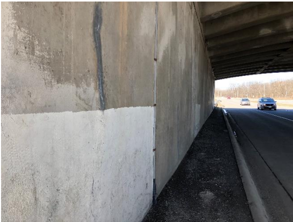
Image 9: Detail of the west abutment, looking north
