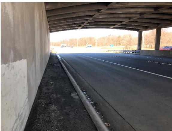
Image 7: View northwest beneath the subject bridge
