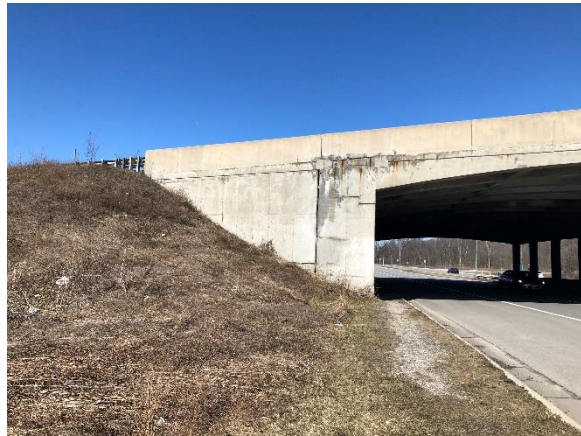
Image 4: View north of the southwest abutment
