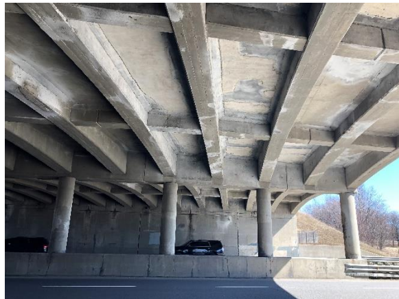
Image 6: Detail of the bridge soffit from underneath the structure
