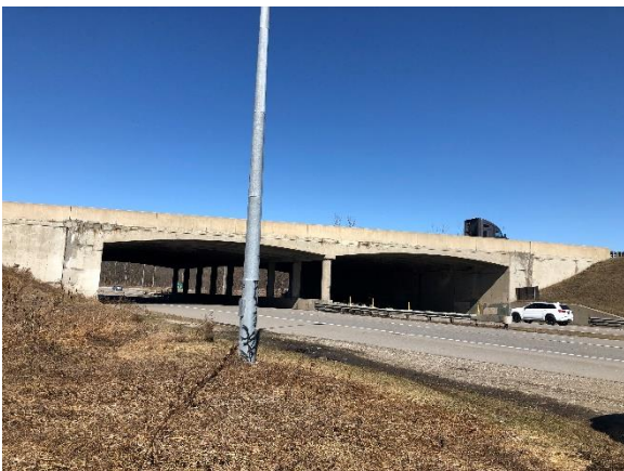
Image 1: Views northwest to the south elevation
