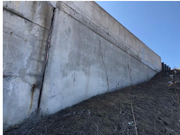
Image 10: Detail of the west abutment, looking southwest
