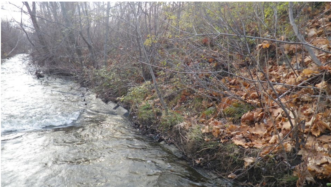
14. Mill Creek Reach MC-1 facing downstream, north of Kerr Street; tiles are lining the bed and banks through the reach (southwest).
