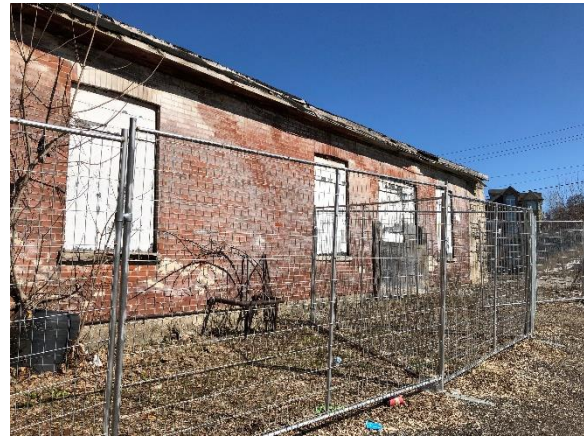
Image 13: View of the south side elevation, 69 Ainslie Street South, looking north.
