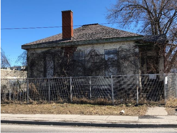
Image 3: Front elevation, 69 Ainslie Street South, Cambridge, ON.
