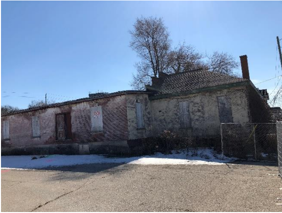
Image 14: View of the north side elevation, looking south.
