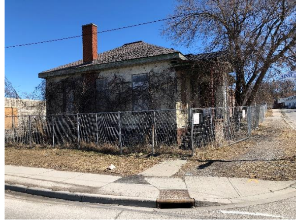
Image 4: Front and south side elevation, 69 Ainslie Street South, Cambridge, ON.
