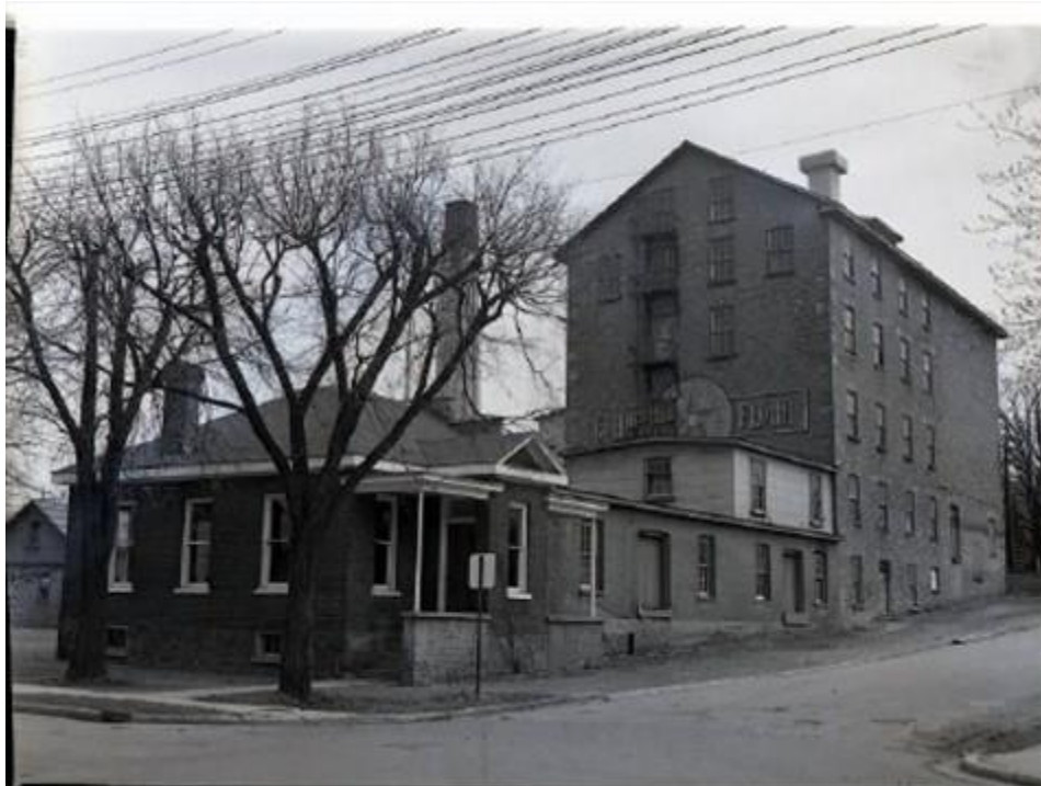
Figure 4: Photograph of Phenix Milling Corp Limited, 1947
