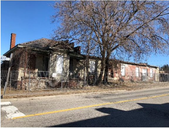
Image 10: View of the south side elevation, 69 Ainslie Street South, looking north.
