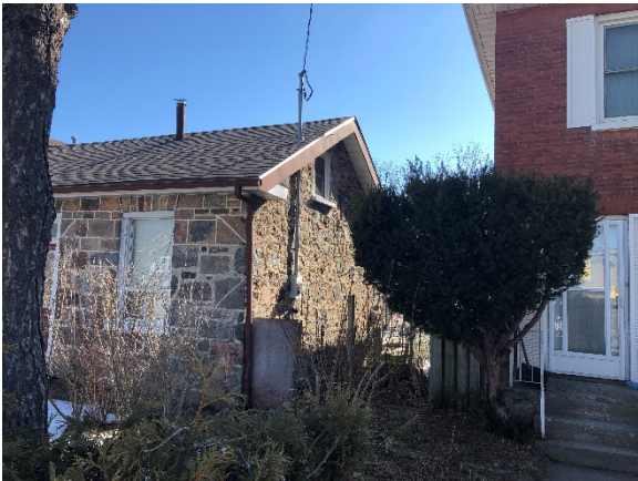
Image 13: View of the south side elevation, looking north.
