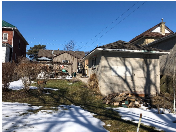
Image 10: Looking northwest towards the rear elevation of 127 Beverly Street from public walking path.
