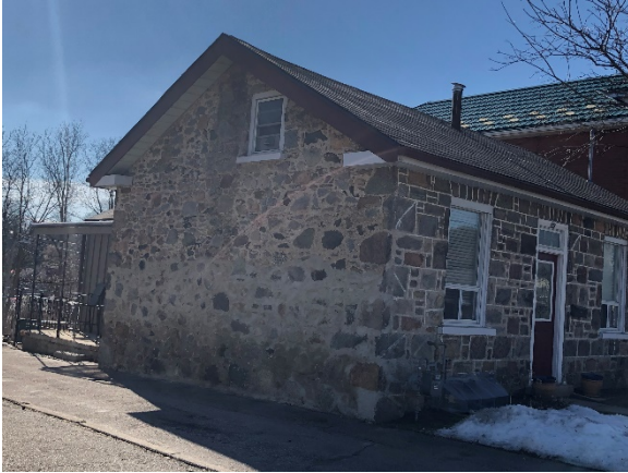
Image 11: View of the north side elevation, 127 Beverly Street, looking southeast.
