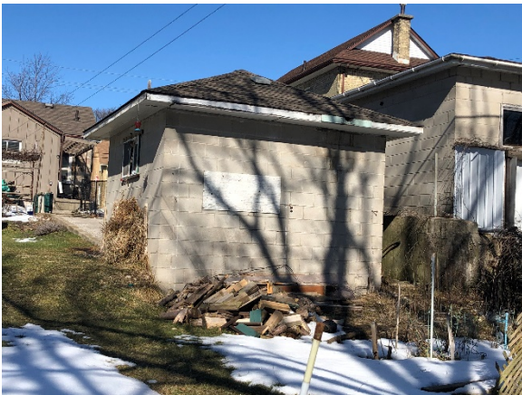
Image 17: Looking northeast towards front elevation of garage structure.
