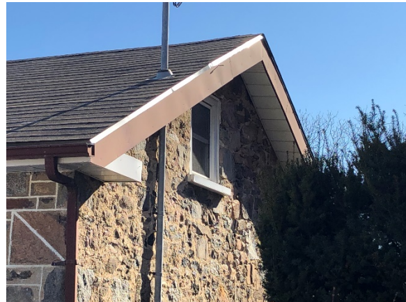
Image 14: View of the side gable, looking north.
