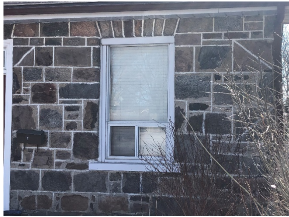
Image 8: Detail view of window opening, 127 Beverly Street, Cambridge, ON.
