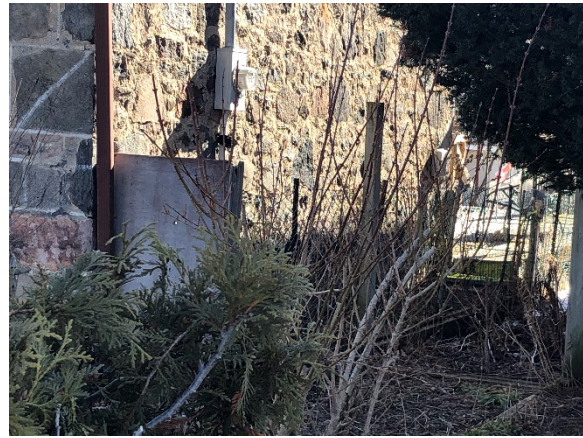
Image 16: View of stone foundation, looking north.
