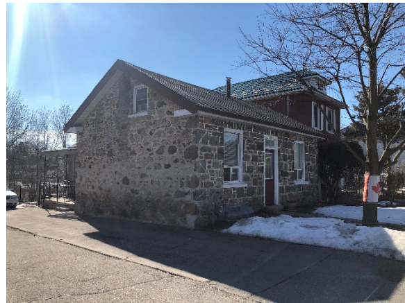
Image 6: Front and south side elevation, 127 Beverly Street, Cambridge, ON.
