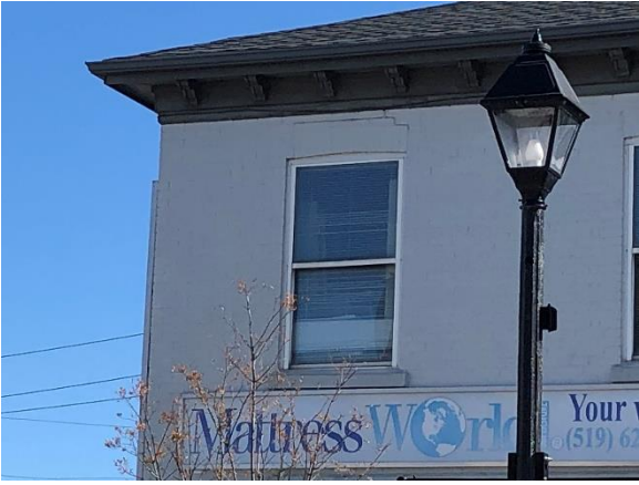
Image 13: View of a second storey window.
