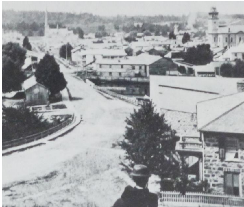
Image 1: View west along Main street from Centennial Park, 1892 (McLaughlin, 1987).
