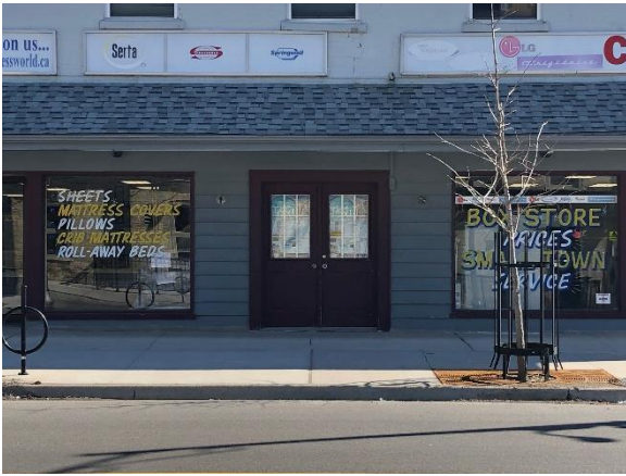
Image 10: View of central doorway.
