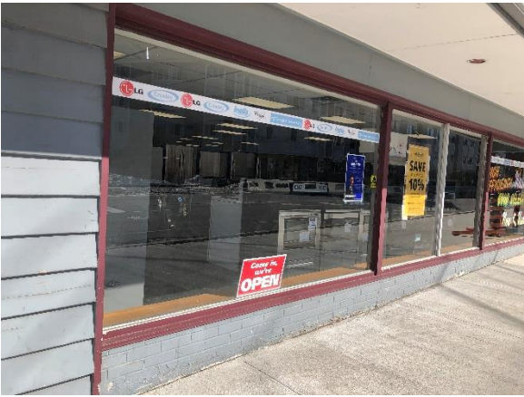
Image 23: View of first storey of south elevation.
