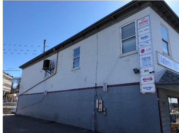
Image 19: View of north elevation.
