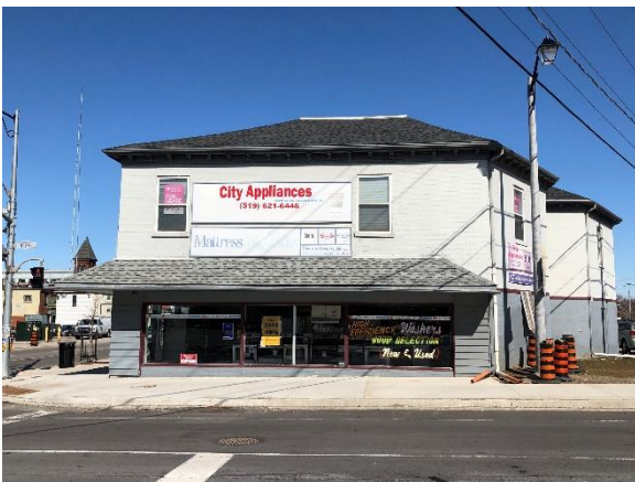
Image 20: View north of the south elevation.
