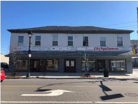
Image 8: View east of front elevation.
