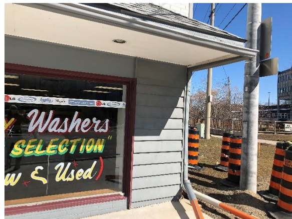
Image 21: View of siding and storefront window.
