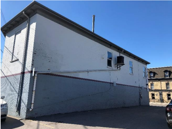
Image 18: View of north elevation.
