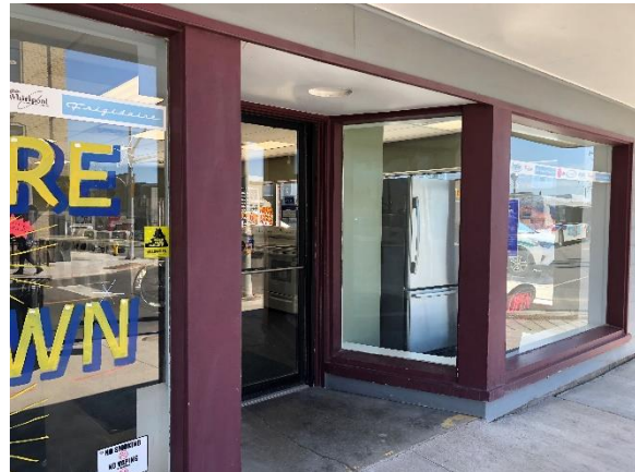
Image 9: View southeast of storefront window details.
