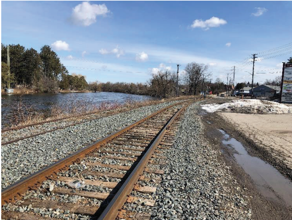
Image 3: View of the existing rail line along Eagle Street, looking easterly.
