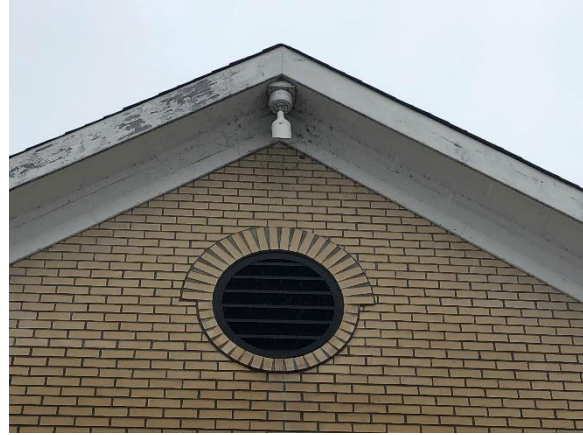
Image 6: Detail of circular vent opening
