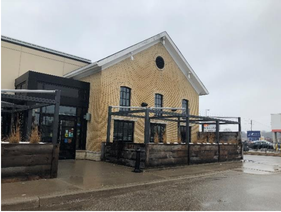
Image 5: View of rear elevation of restaurant at 4336 King Street East
