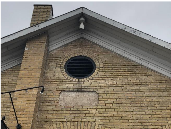
Image 9: Detail of gable end, note wood cornice, circular vent and inset panel
