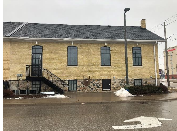
Image 12: View of the west side elevation of the former Pine Grove Schoolhouse
