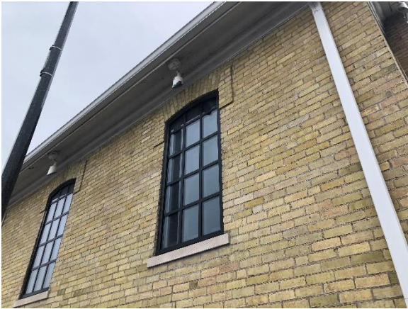
Image 17: View of window opening on the west side elevation
