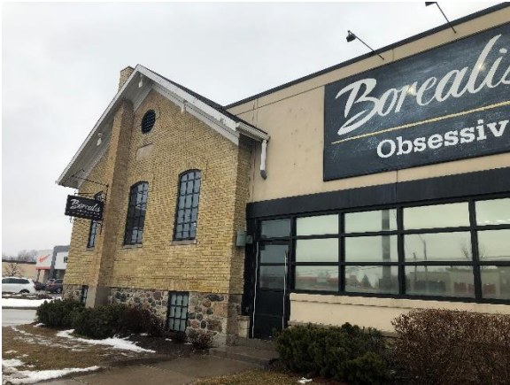
Image 7: View of the front elevation of 4336 King Street East
