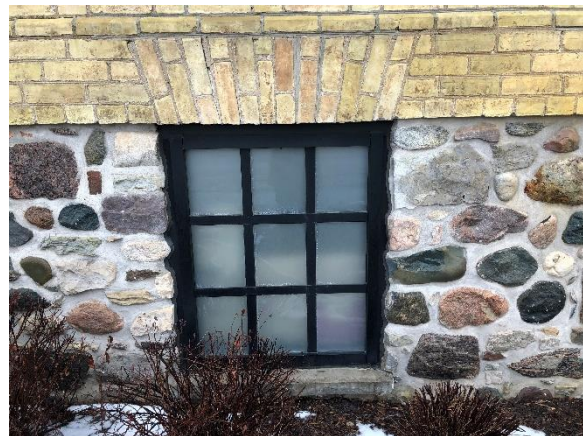
Image 10: Detail of basement window opening
