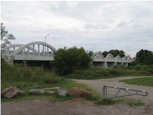
Freepoint Bridge (ARA Architects, Sep. 2015)
