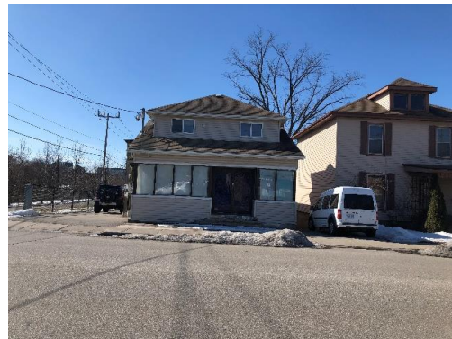
Image 6: Front elevation, 41 Kerr Street, Cambridge, ON.
