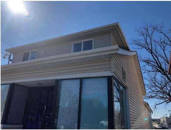
Image 7: Detail view of covered porch, entranceway, and second storey addition, 41 Kerr Street, Cambridge, ON.
