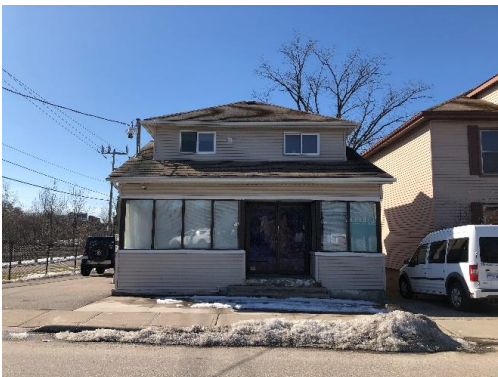
Image 5: Front elevation, 41 Kerr Street, Cambridge, ON.
