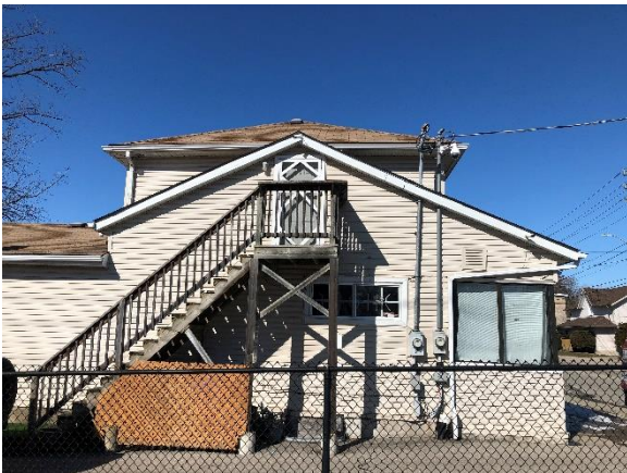
Image 13: View of the east side elevation, 41 Kerr Street, looking southeast.
