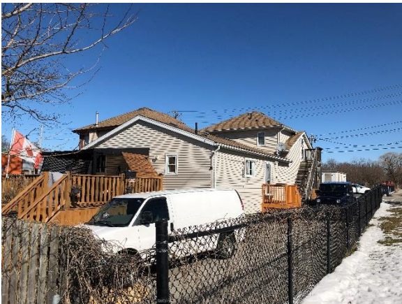
Image 9: Looking northwest towards the rear elevation of 41 Kerr Street from public walking path.
