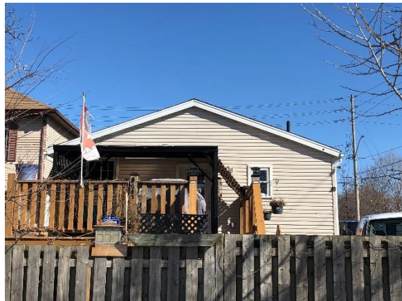
Image 10: Looking north towards the rear elevation of 41 Kerr Street from public parking lot.
