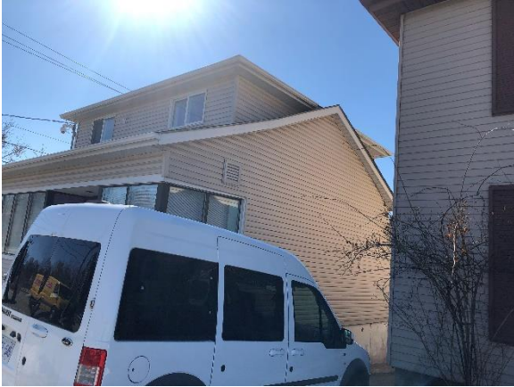
Image 15: View of the west side gable, looking east.
