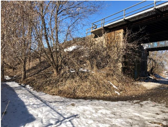
Image 1: View towards the southwest corner of the bridge and west approach.
