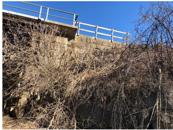
Image 3: View of the east stone abutment and retaining wall, looking north.
