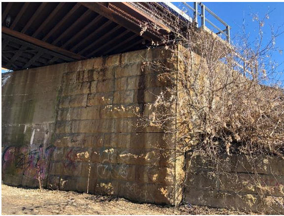
Image 2: View of the east stone and concrete abutment.
