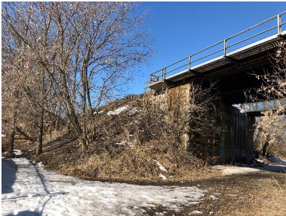
Image 4: View of the west stone abutment.
