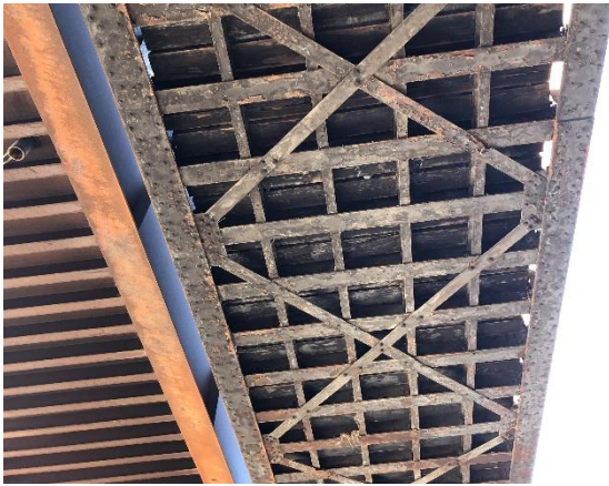
Image 14: Detail of soffit of middle bridge deck.
