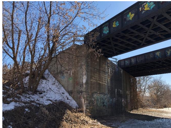
Image 7: View of the east concrete abutment, looking south.
