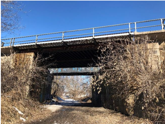
Image 10: View of the bridge decks.
