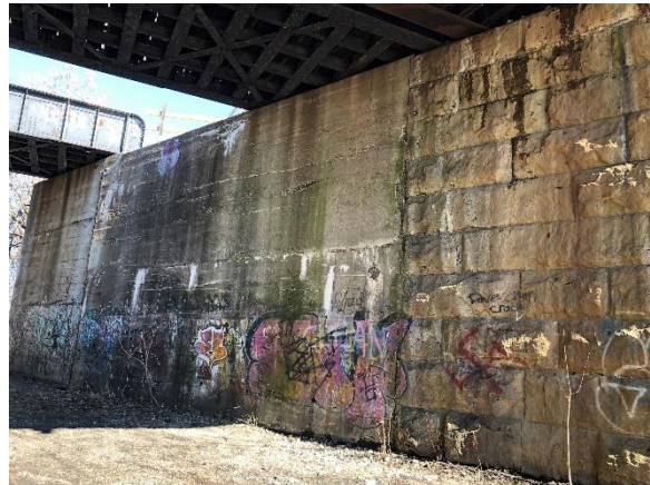
Image 5: Full view of the east abutment.
