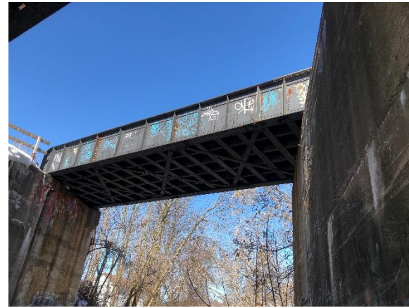
Image 15: View of north bridge deck.
