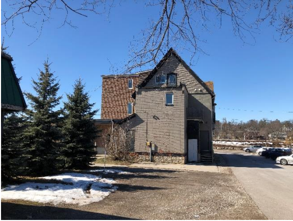
Image 10: View of the rear elevation including the former dwelling and two-storey rear addition.
