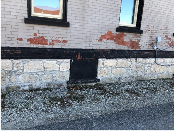
Image 16: Detail of a basement window opening on the north side elevation.
