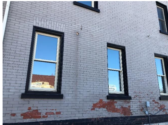
Image 15: Detail of first storey window openings on the north side elevation.
