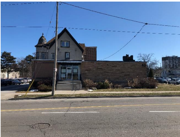
Image 4: View of front (west) elevation.
