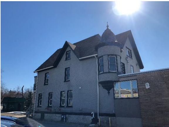
Image 14: View of the north side elevation.
