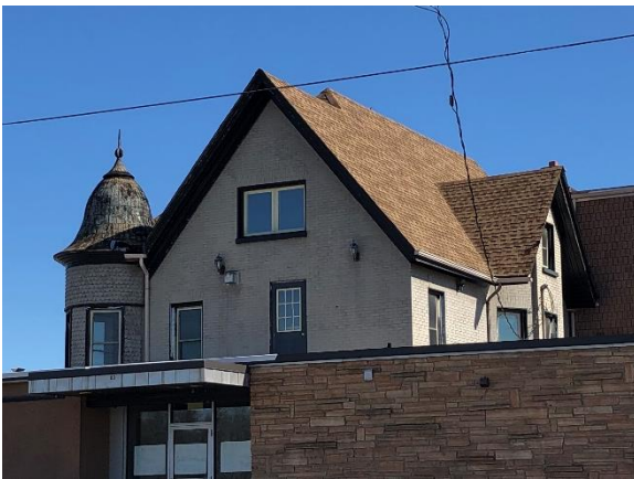
Image 6: View of the second-storey façade
