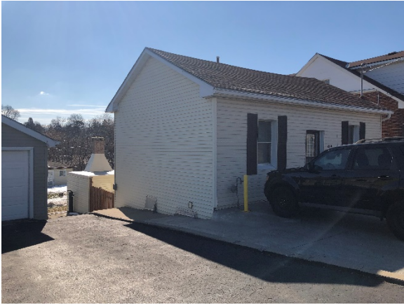
Image 13: View of the north side elevation, 99 Beverly Street, looking southeast.
