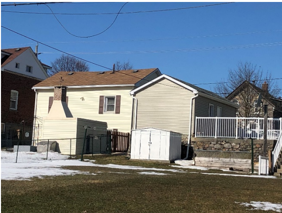
Image 18: Looking northwest towards rear elevation of garage structure and house.
