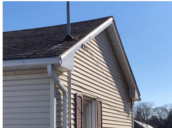
Image 16: View of the side gable, looking east.
