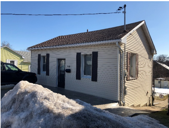
Image 15: View of the south side elevation, looking east.
