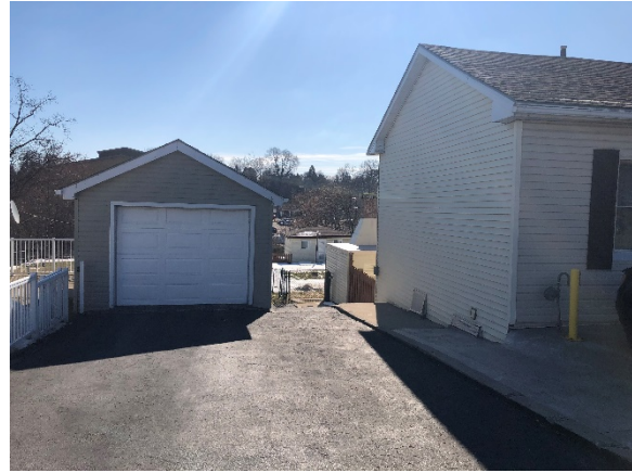
Image 14: View of the north side elevation, 99 Beverly Street, looking southeast.
