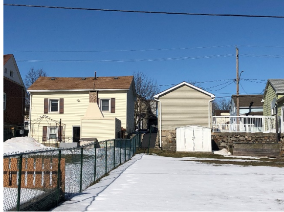
Image 10: Looking northwest towards the rear elevation of 99 Beverly Street from public walking path.
