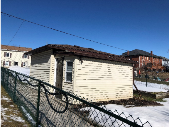
Image 20: Looking northwest towards rear shed structure.
