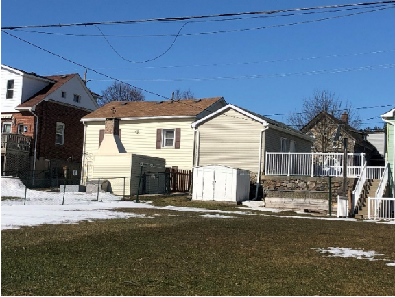
Image 9: Looking west towards the rear elevation of 99 Beverly Street from public walking path.
