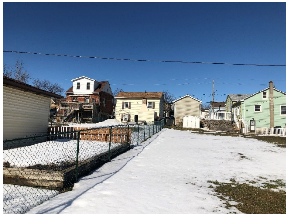
Image 12: Looking northwest towards the rear elevation of 99 Beverly Street from public walking path.
