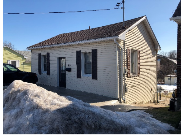
Image 6: Front and south side elevation, 99 Beverly Street, Cambridge, ON.
