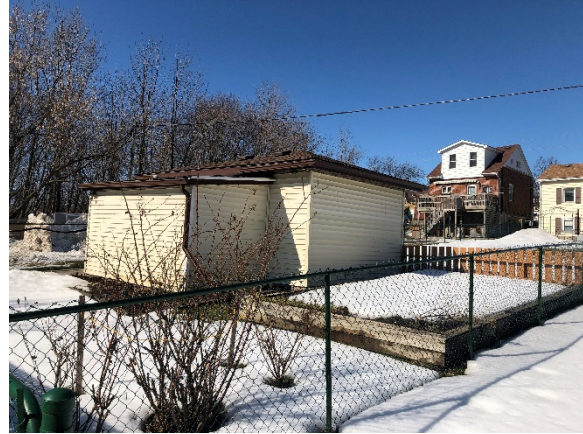
Image 21: Looking southwest towards rear shed structure.
