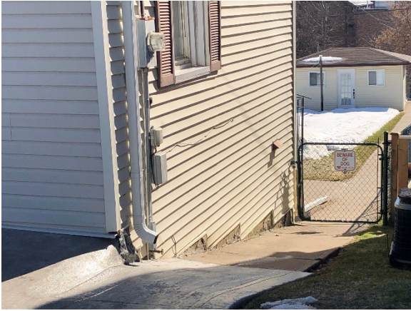
Image 17: View of the foundation, south side elevation, looking east.
