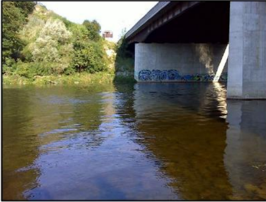
Grand River: View of proposed LRT crossing location from the south bank.
