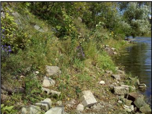
Speed River: West bank showing existing fill (at proposed LRT crossing area).
