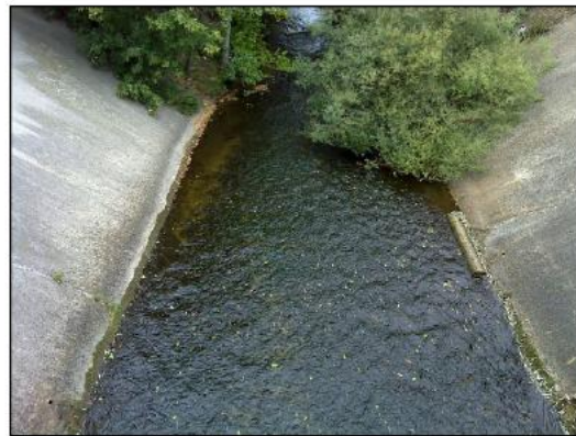
Mill Creek: Upstream view from near Main Street (concrete trapezoidal channel).
