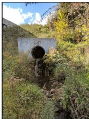
Hofstetter Creek culvert outlet (perched).
