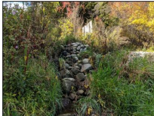
Hofstetter Creek outlet to the Grand River (Fall 2018).
