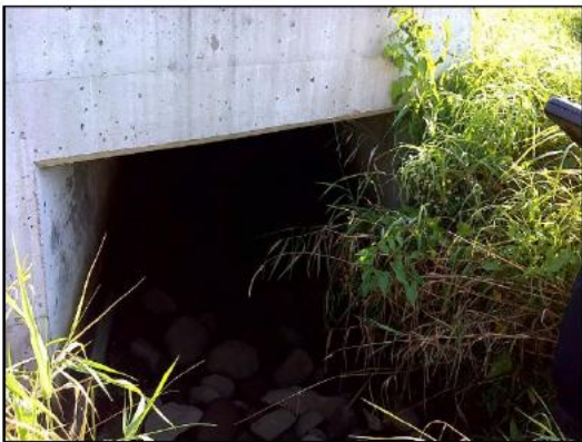
Freeport Creek: Highway 8 culvert outlet.
